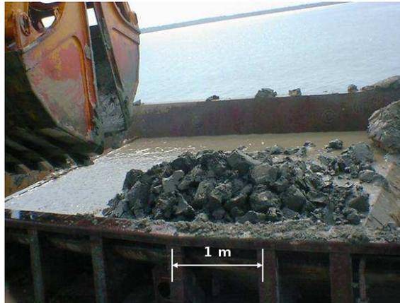
FIGURE 1. View of dredged clay lumps placed in a barge before dumping in the sea
